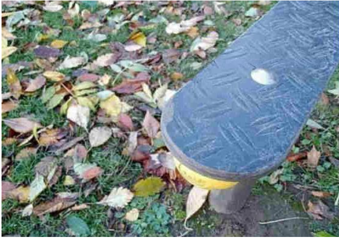
Figure 1: Wear on balance Beam (Very Low)
